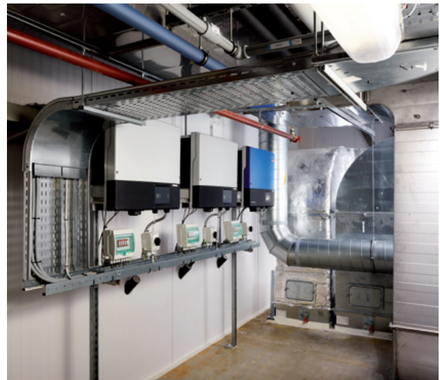
Real installation situation
